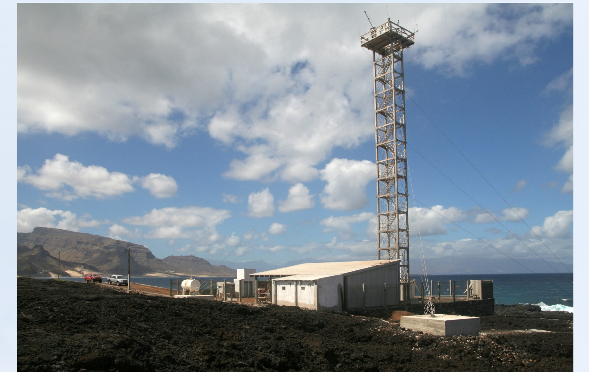
Fig. 1. Cape Verde Atmospheric Observatory (CVAO) with a 30 m-tower for aerosol particle sampling, ~100 m offshore.
