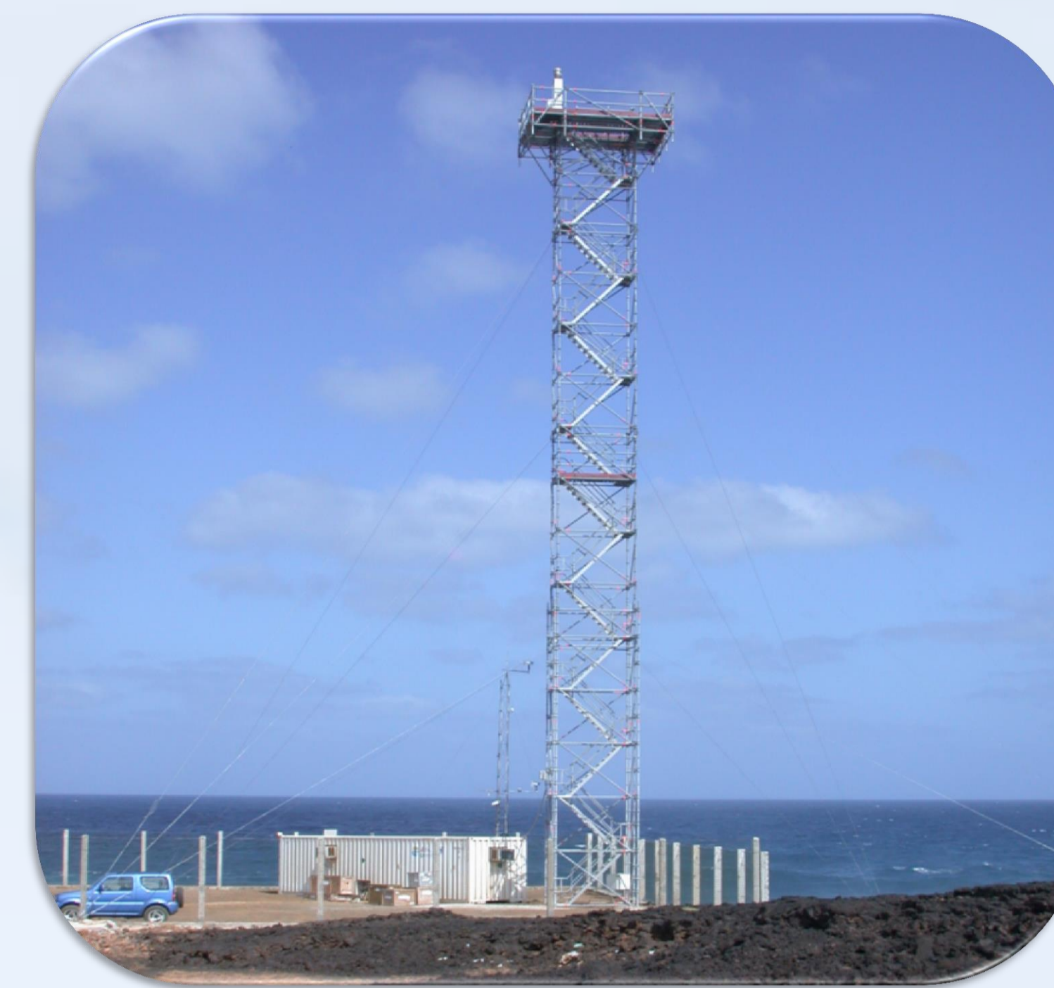
Fig. 1: Cape Verde Atmospheric Observatory (CVAO) with a 30 m-tower for Aerosol particle sampling, ~100 m offshore.
