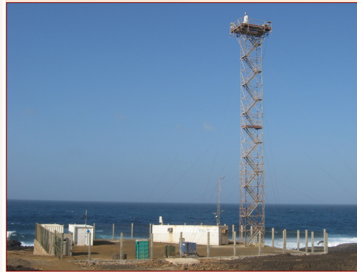
Fig. 2: Atmospheric observatory with 30 m-tower for chemical measurements, ~100 m onshore
